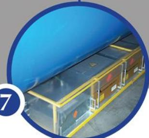
6500 new detectors are being added to the magnet protection system, requiring 250 km of cables to be laid
