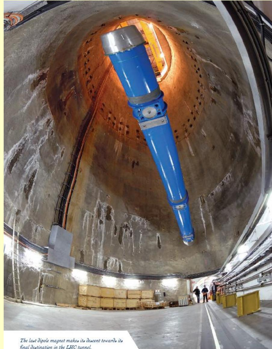
*The last dipole magnet makes its descent towards its final destination in the LHC tunnel.*
