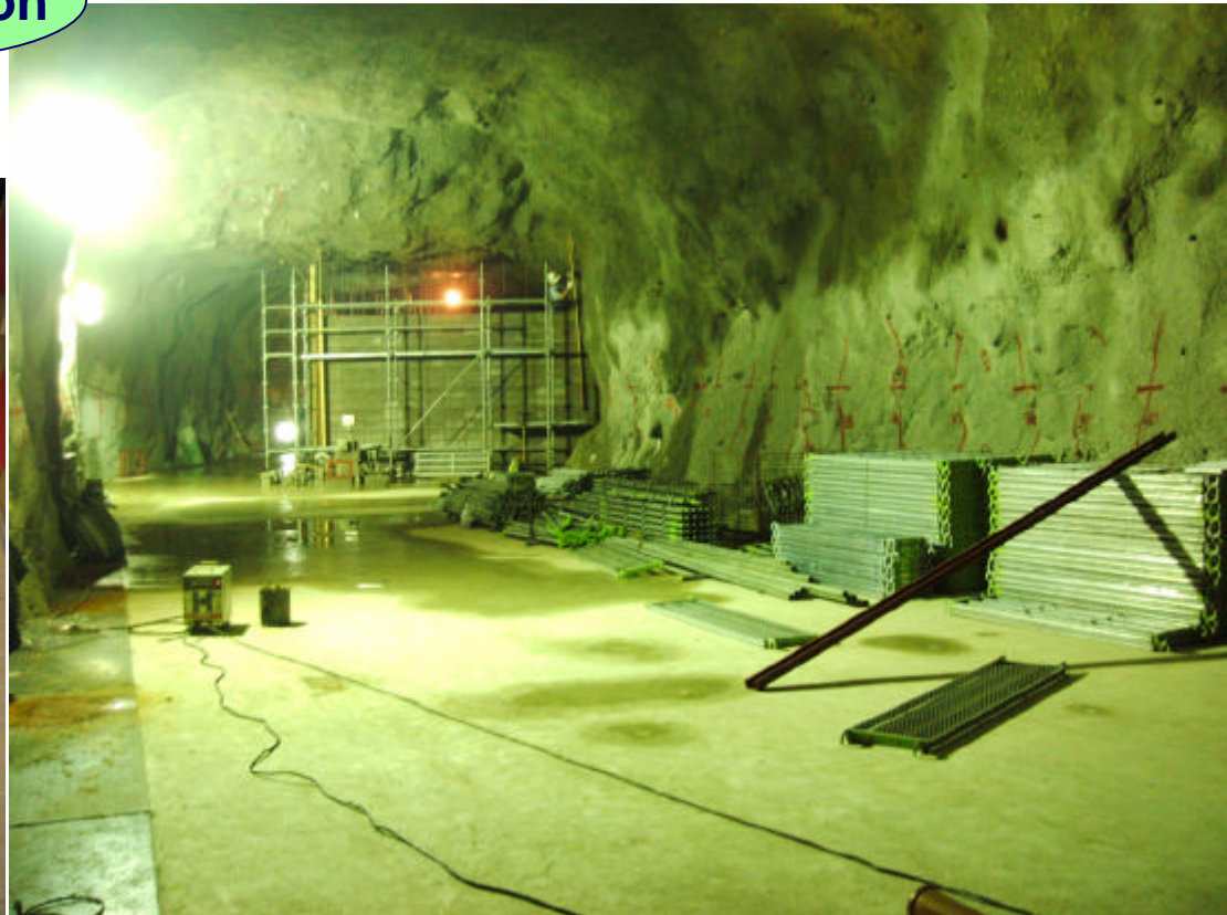
New tunnel for the purification system
