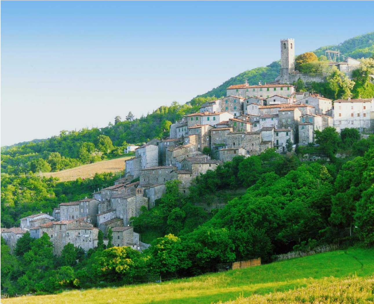
Castelnuovo District Heating - Italy
