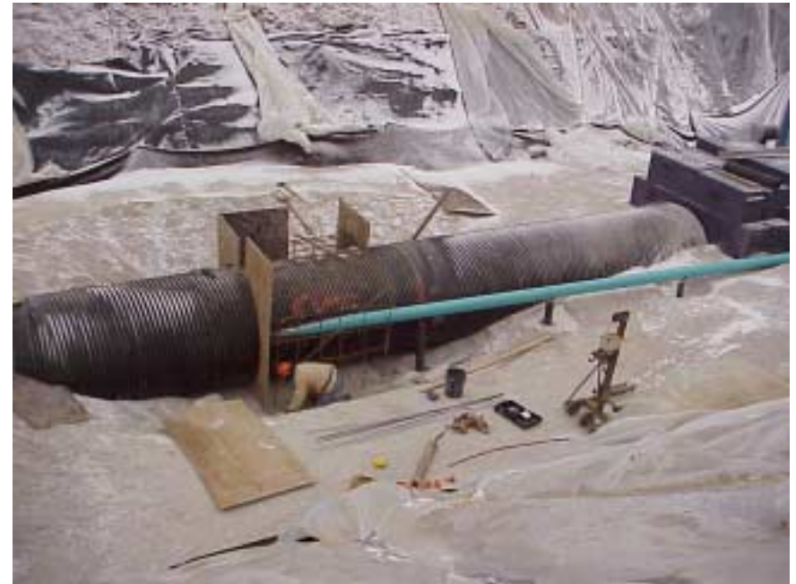
The LMC drift pipe during construction
